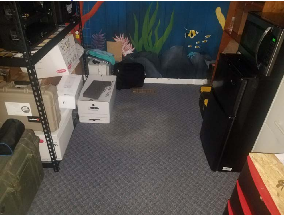
Carpet applied to concrete. Not a suspect asbestos containing material (ACM).
