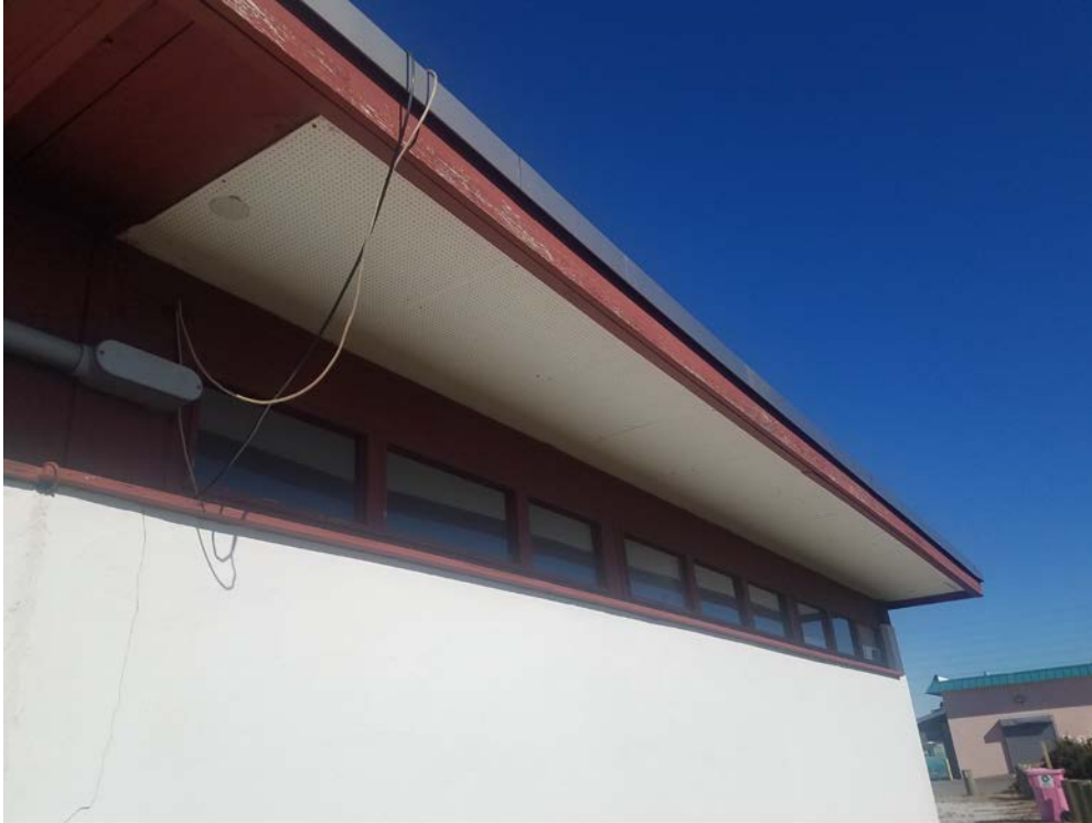
HM-05: Transite® paneling applied to eaves.
