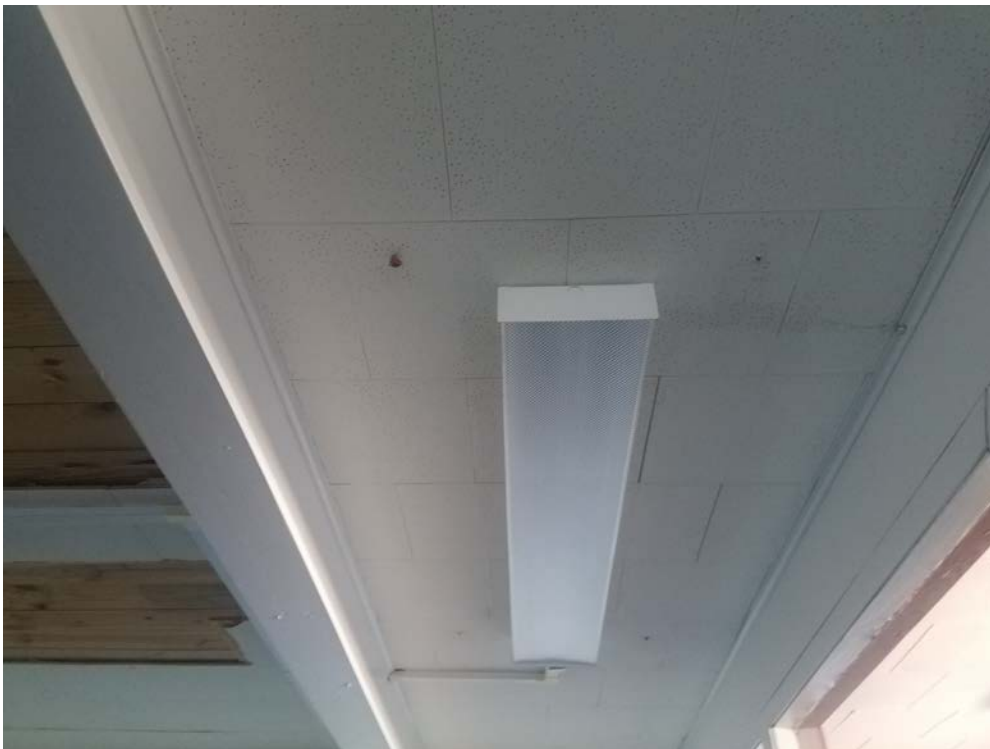
HM-01/HM-02: 12" Ceiling Tile applied in various room areas. Non-asbestos.
