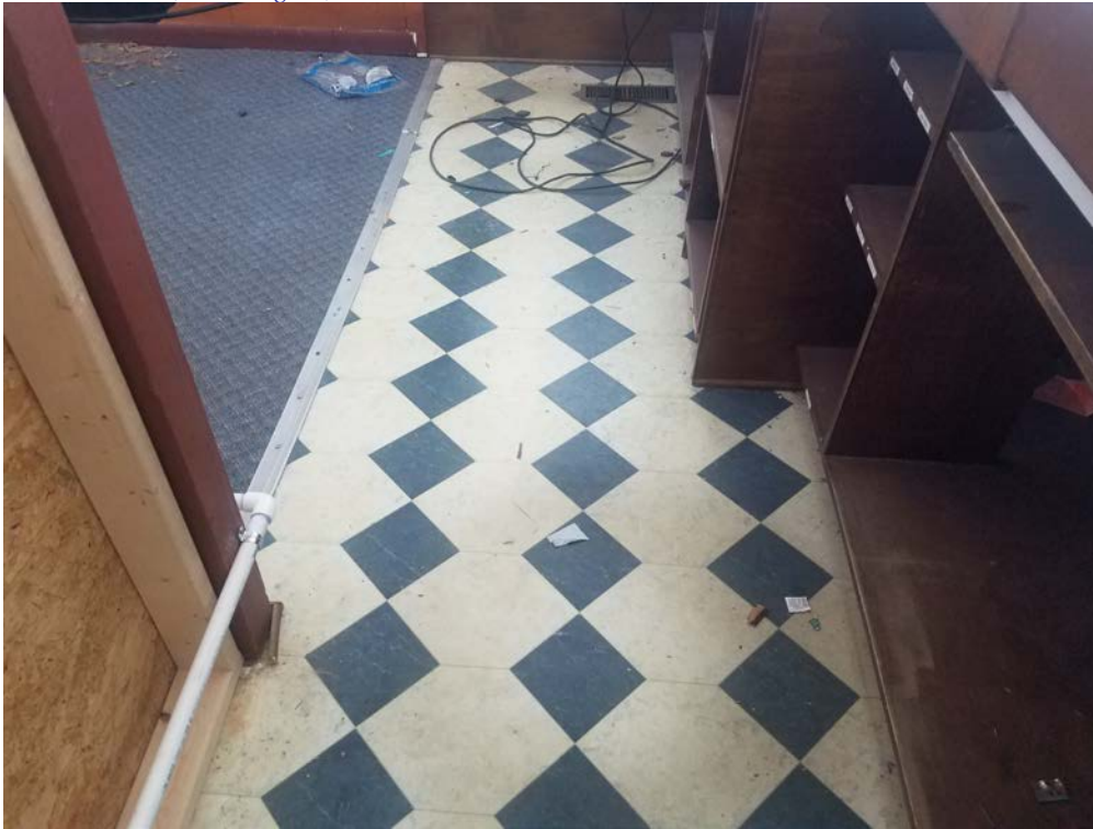
HM-06: Linoleum (Blue/Green/White). Applied in one additional room. Non-asbestos containing material.
