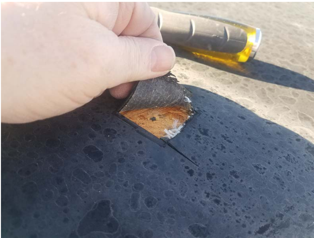
Rubberized Roof over Plywood. Not a Suspect ACM.
