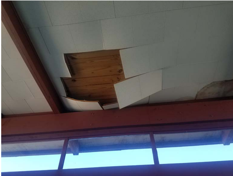
12" Ceiling Tile. Cellulose Backed. Not a suspect ACM.
